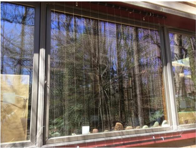
Here's the back-yard window, from the outside in. You can see the way it's put together (look at the bottom-right corner). Just one screw per (four) holding-hooks, and then the horizontal bar pops into place, holding the fishing lines taught. Also, the preventer is easy to remove or reposition to wash the windows.
